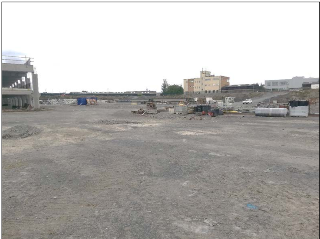
Plate 2.2 Spoil and bare ground (ED2) & existing buildings (BL3) (June 2019)
